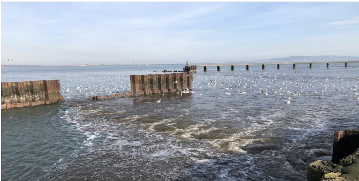
Fig 4.1 Discharge Point – 25 February 2019
